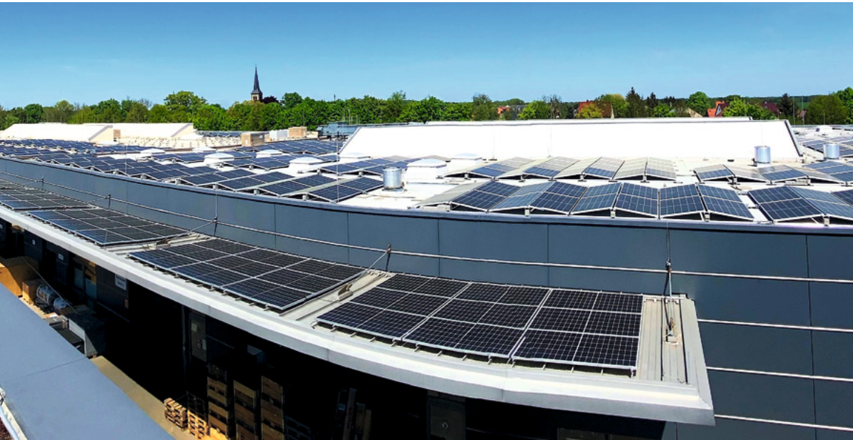
NEW INSTALLATION OF A PV SYSTEM IN 2022 AT OUR SITE IN OTTENDORF-OKRILLA WITH AN OUTPUT OF OVER 500 KWP
