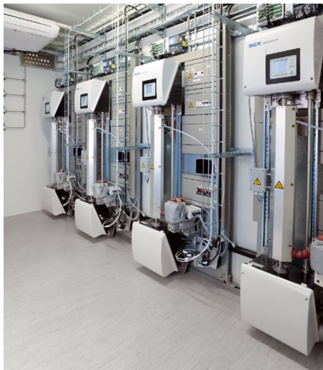
MCS300P: Raw gas measurements in an analyzer container
