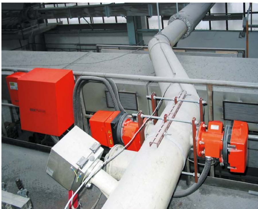
Measurement of ammonia in composting and waste incineration plants – also in hospitals
